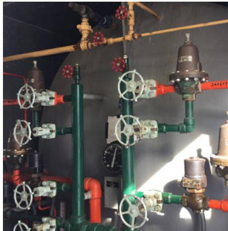
Pressurization plant including a 3,500-gallon storage tank that will be removed as part of the Rochester Airport Cable Refurbishment project.
