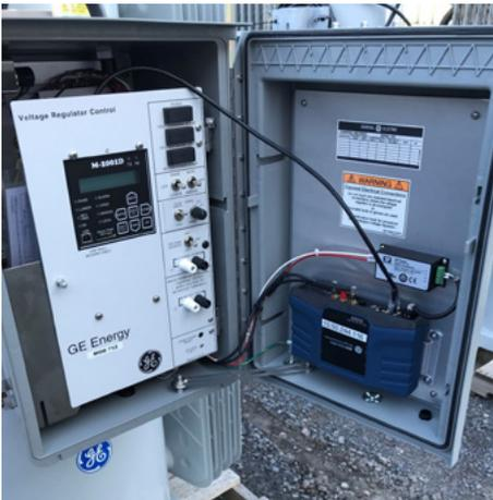
GE control cabinet meant to operate regulators for the Volt-Var Optimization scheme.
